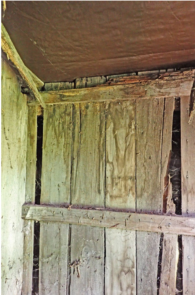
Photo 23 Chinese Bunkhouse, interior detail of boxed frame construction, camera facing east
